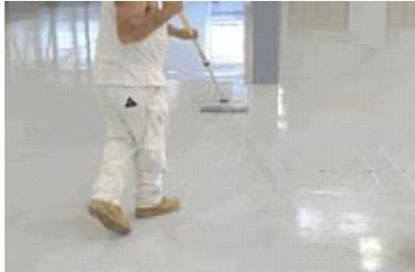
Good ventilation and air movement is essential to assist drying especially in damp atmosphere.
